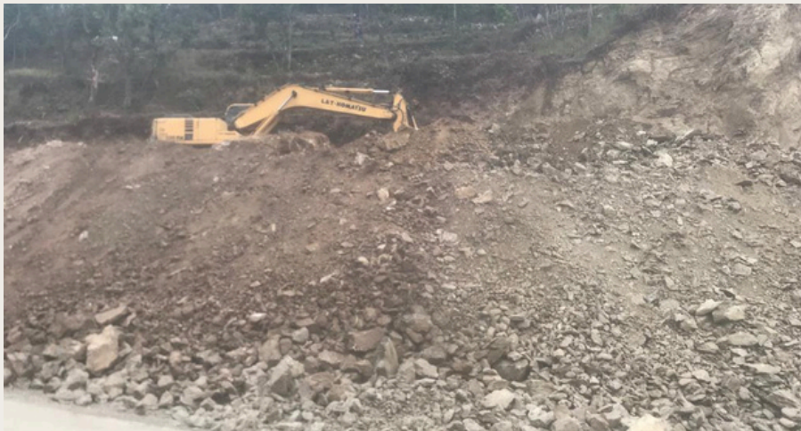
All Weather Road, Kandwali, Risikesh
