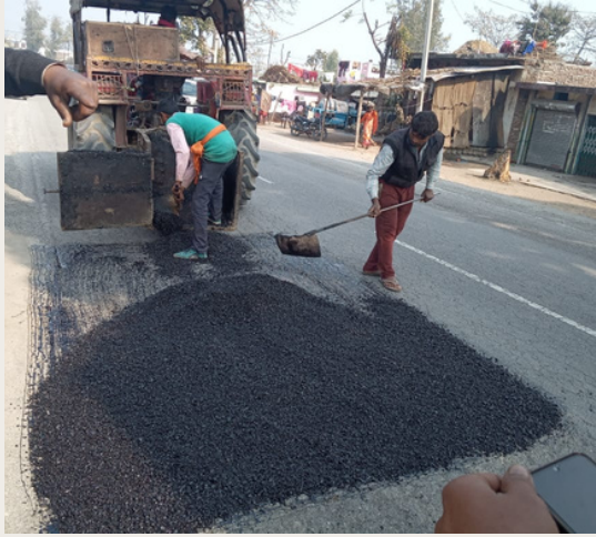
Filling Of Potholes, NH-72
